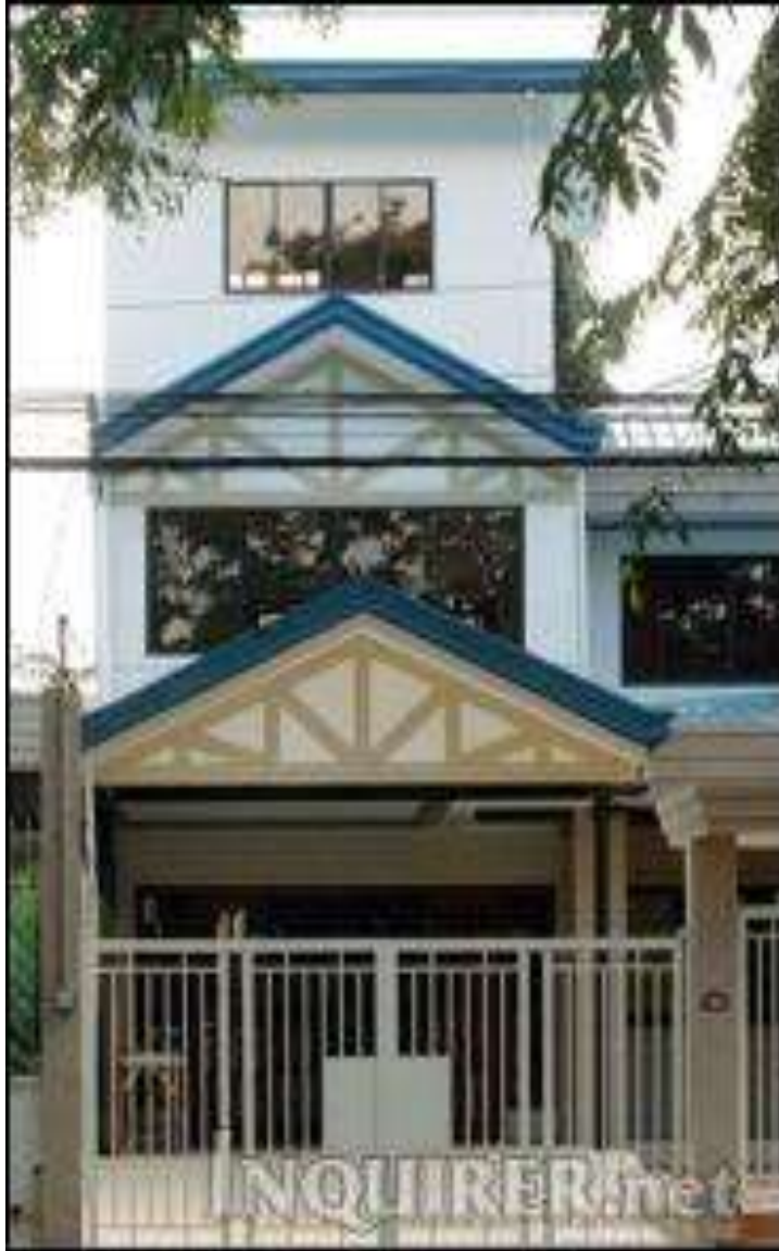
Panic room added in a house in Provident Village, Marikina after Ondoy
