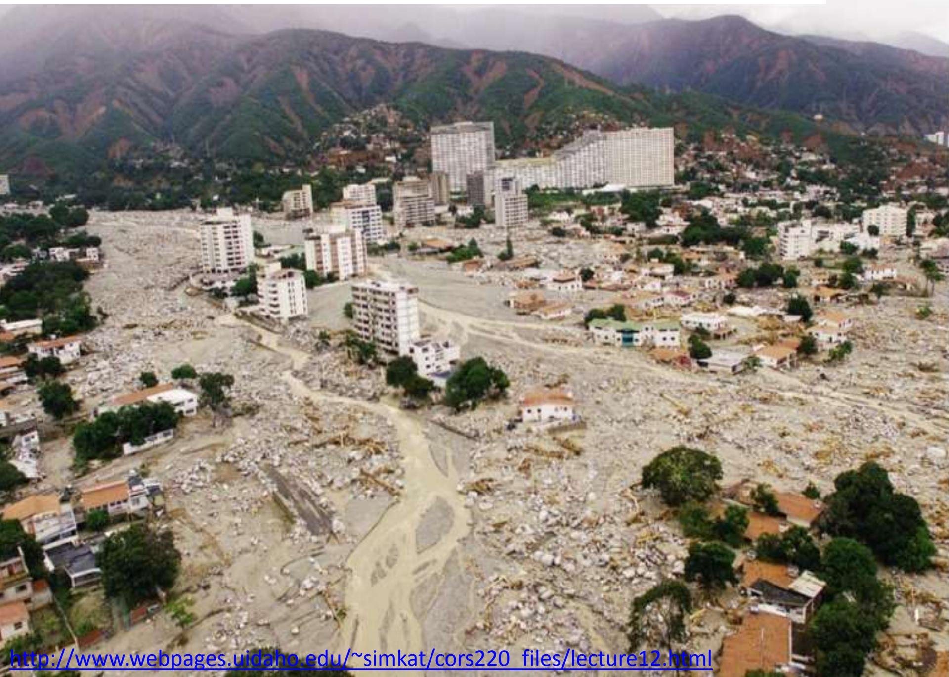
Debris flow field in Cordillera de La Costa, Vargas, Venezuela. 19,000 died in 1999
