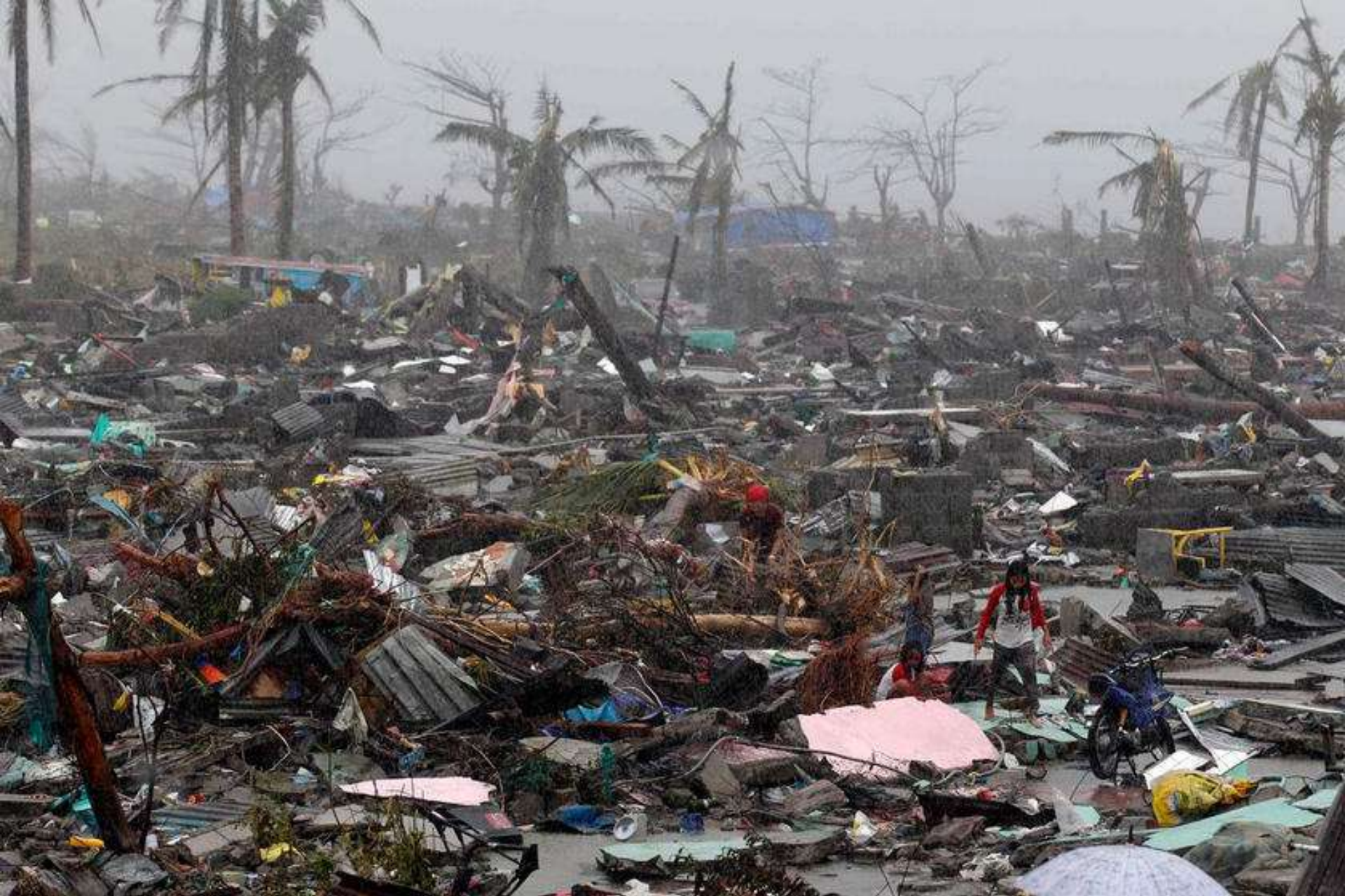
Houses-turned-debris & rubbles in Tacloban City
