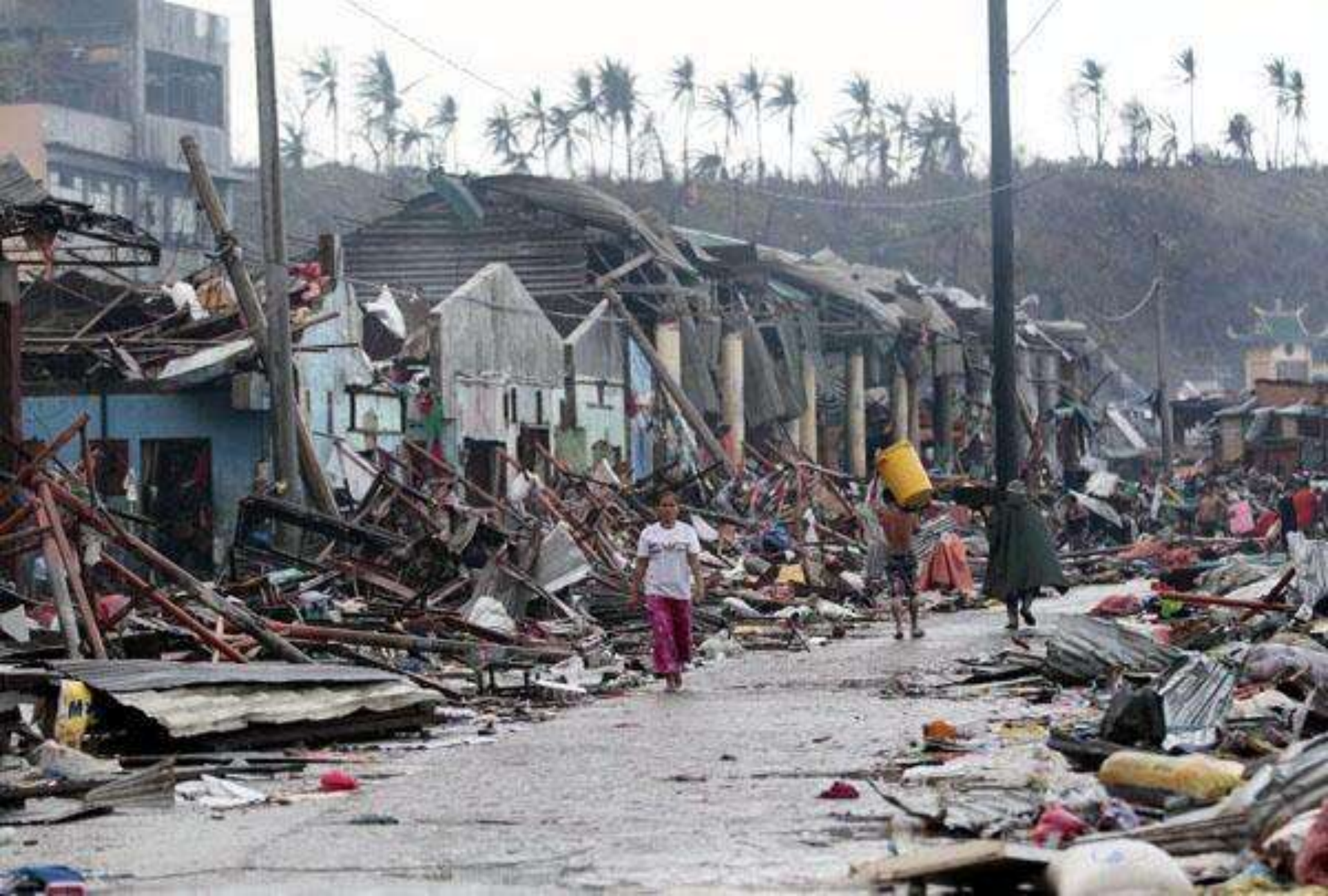
Totally damaged houses in Tacloban City, Leyte
