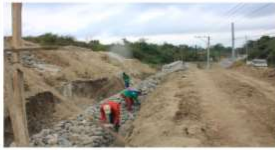
Establishment of Bench Terracing & perimeter fencing
