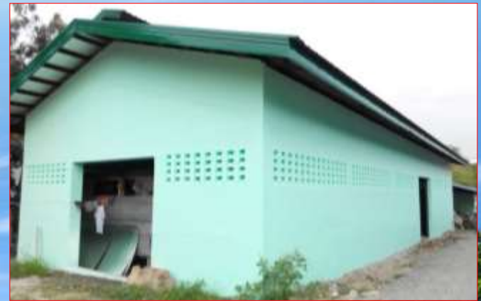
Seeder Machine Building
